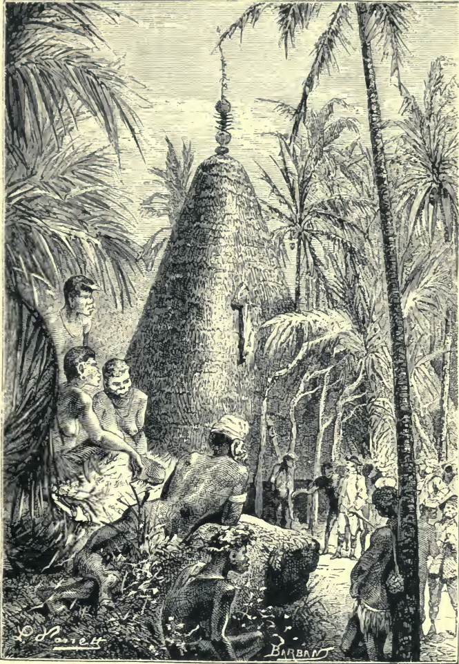
With the roof of considerable height.
